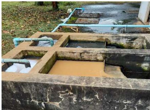
Brownish water indicates heavy stormwater intrusion in an ASP
