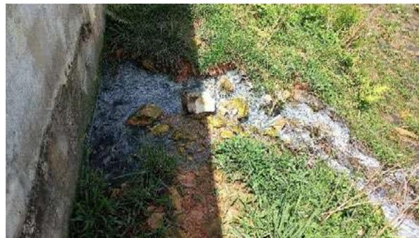
Poor construction quality has led to leakages in the settler, subsequently causing environmental pollution in the adjoining area
