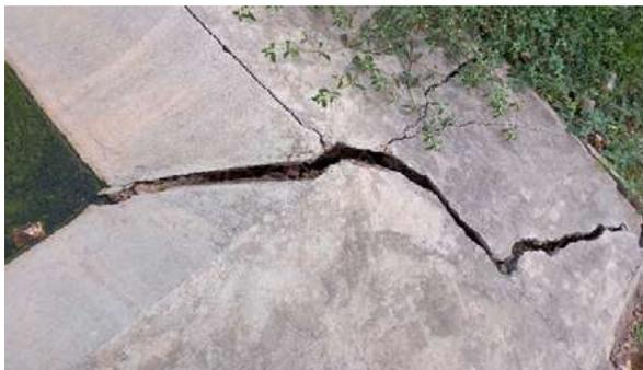
Poor construction quality has led to a broken dam structure in a wastewater pond, thus causing leakage
