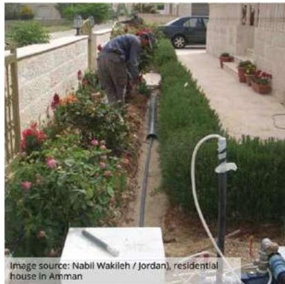
**Figure 6.14.** French drain system
