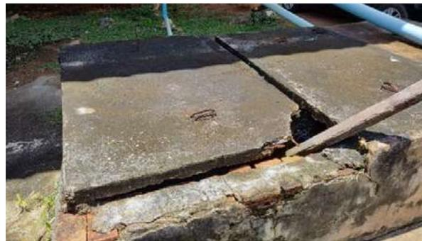
The manhole lids of the collection tank are extremely heavy; hence, it is difficult to maintain the tank and it becomes a source of odour and insects
