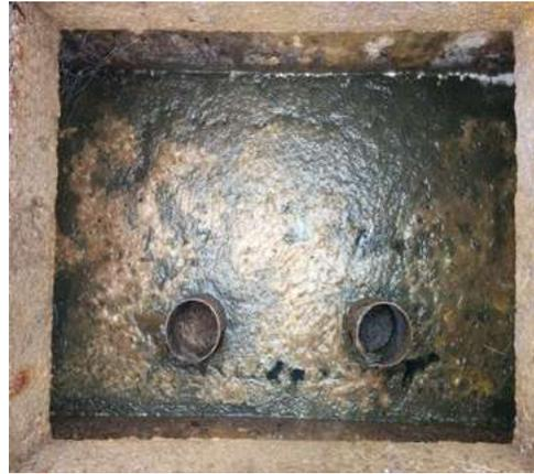
Scum development in an ABR chamber due to a high organic loading rate or due to a extremely high sludge accumulation rate caused by missing regular desludging appointments
