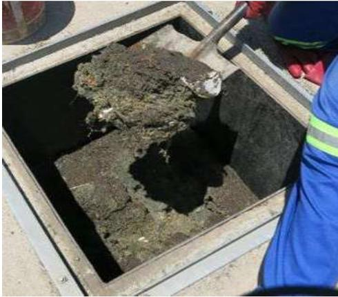
Unusual high scum accumulation in the settler and septic tank; in this case, this is due to a very high grease concentration in the incoming wastewater.
