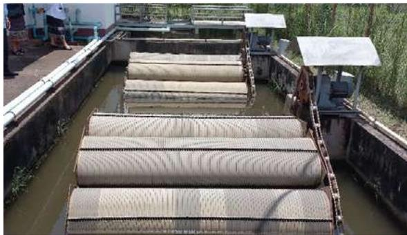
In a rotating disc contactor, the reactor surface is dry and without bio-film; thus, the disc is not operational, resulting in no treatment
