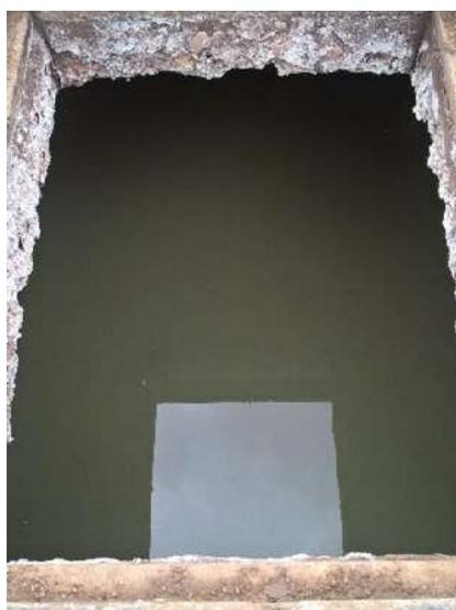
Yellowish and whitefish accumulation and dissolving concrete surface indicate ineffective ventilation of an anaerobic tank (settler, septic tank, ABR, AF) and the presence of sulphurous gases in the wastewater.
