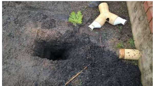
This is the same constructed wetland as that in the photo to the left, after removal of the pounding water and plants. The blackish sand indicates unwanted anaerobic zones and deep organic sludge penetration into the sand filter. This is caused due to overloading and long-term pounding of water.
