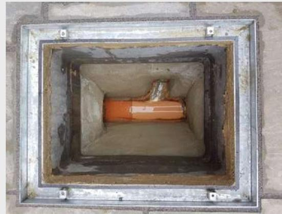
**Figure 4.15.** Brick- built manhole
