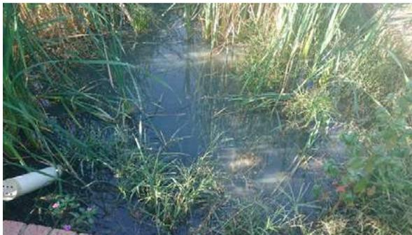
Pounding wastewater in a vertical flow constructed wetland indicates that the wetland is clogged and has lost its infiltration capacity
